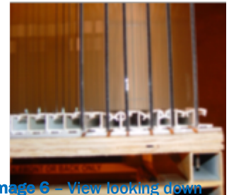
Image 6 - View looking down at gasket with glass inserted.
