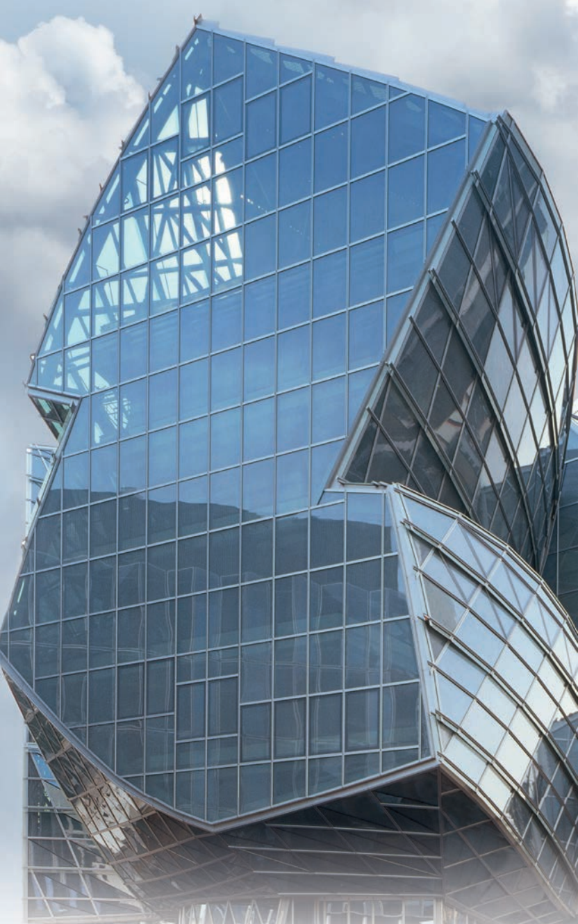
Novartis Gehry Building, Basilea, Suiza | SunGuard® HP Neutral 60/40 Arquitecto: Gehry Partners LLP | Foto: © Hans Ege
