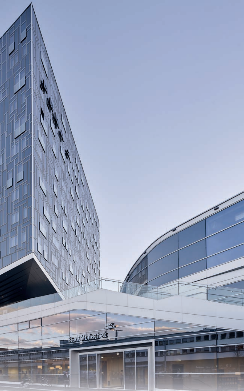
PEMA II, Innsbruck, Austria | SunGuard® HD Light Blue 52 Arquitecto: LAAC | Foto: © Marc Lins
